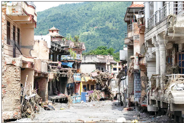
A street looks deserted following a flash flood in Devighat village, Nuwakot district, Nepal on Friday.
