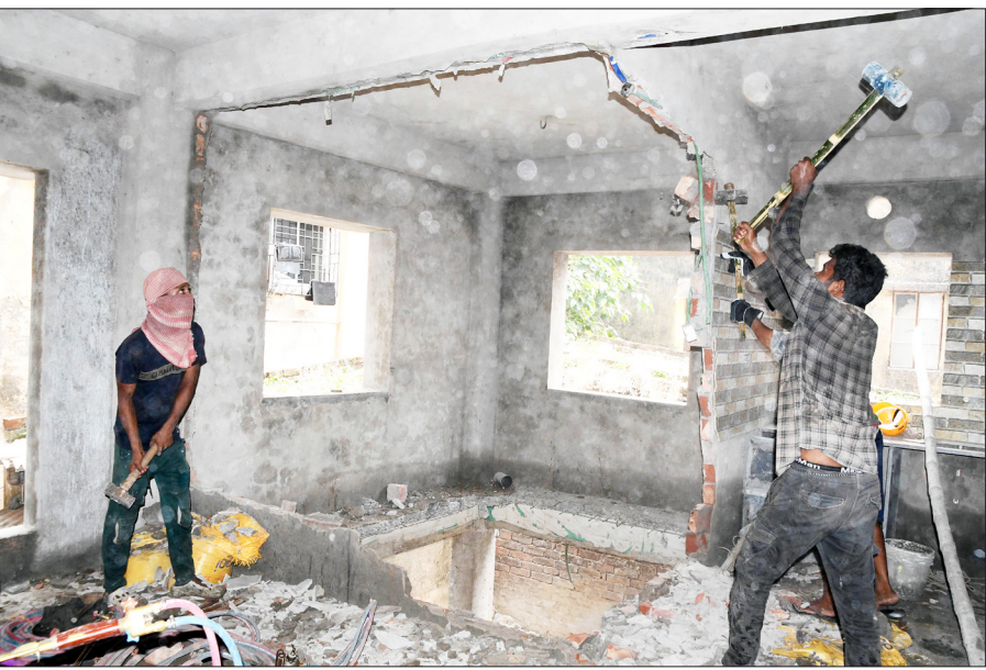
A building developed by Sona Pappu at 142 B.B. Chatterjee Road in Kasba is being demolished by the Kolkata Municipal Corporation (KMC) on Sunday.
