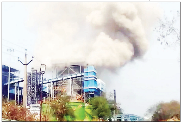
inside the plant at the time of the incident. Following the explosion, pandemonium ensued as everyone scrambled simultaneously to flee the facility in a desperate bid to save their lives; this chaotic rush led to a stampede-like situation. As of now, nine fatalities have been
